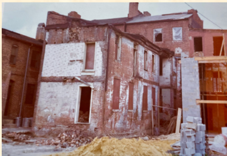
Pre-renovation view of the rear of 113 W. Lee
