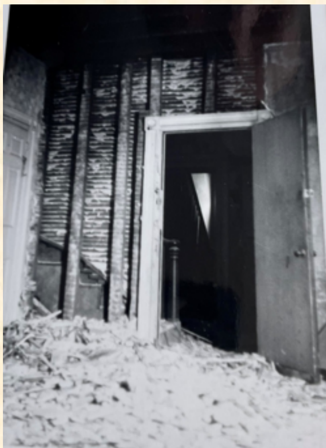
Imagine the possibilities as demolition proceeds!
