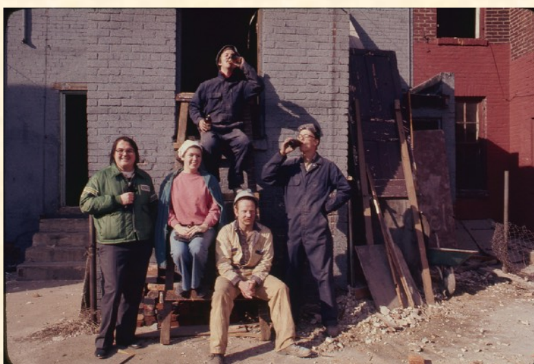
Rehab crew on break, with Steve on the right.
