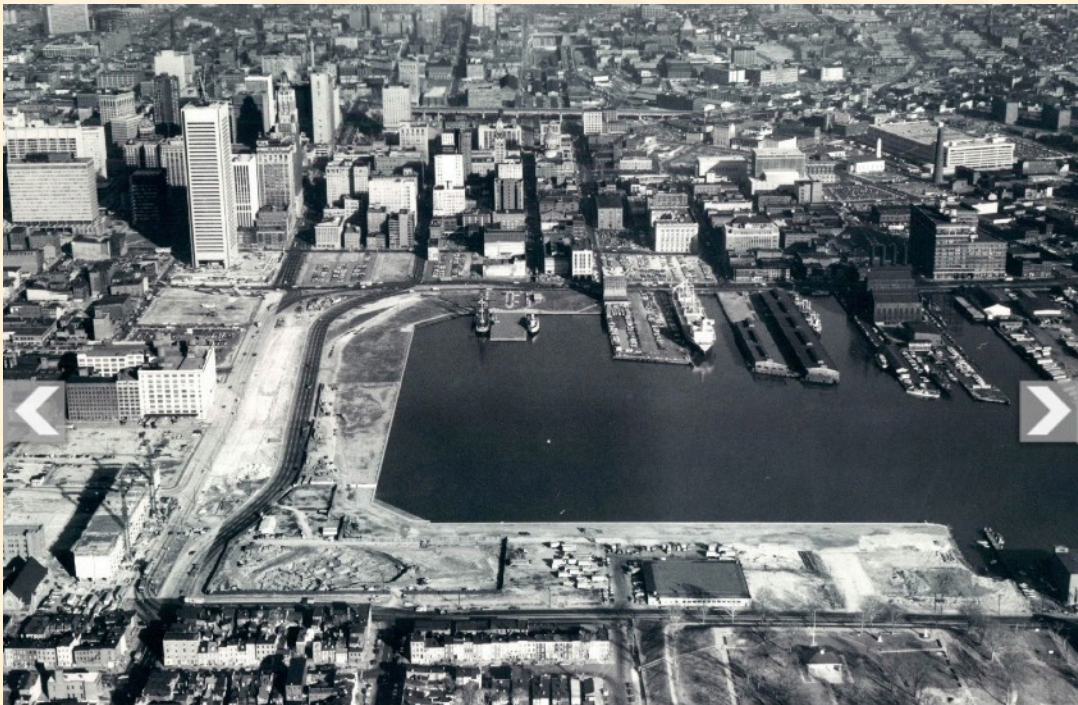
Inner Harbor under construction, 1973
